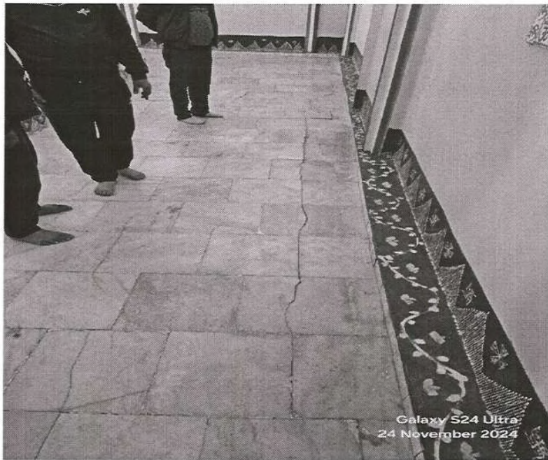
Photo 3- Cracks in flooring of Kalika Temple
